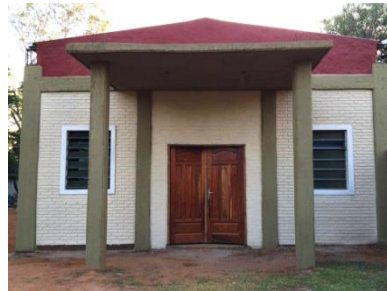
The façade at Barrio Parque. Note the new door, windows and newly completed stucco and paint.
