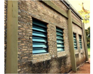
New windows installed at Barrio Parque.
