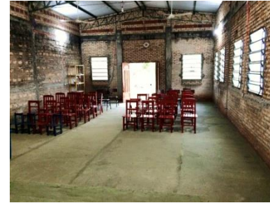
A new concrete floor at Barrio Parque!
