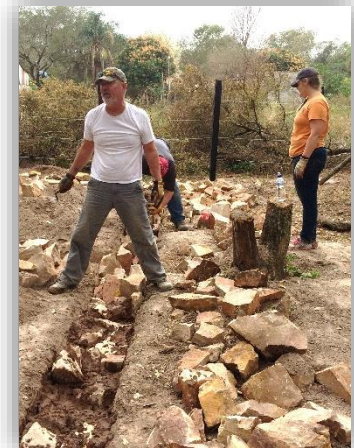
Construction on building foundation at Marin.
