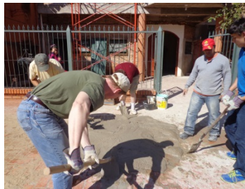
Mixing concrete for the stucco on the outside walls
