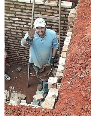
Pastor Miguel and his crew are diligently working on the new septic tank for Barrio Parque Church. The previous was destroyed during torrential rains.
