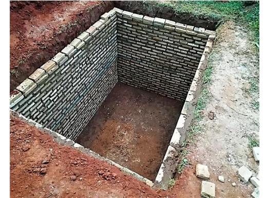
Pastor Miguel and his crew are diligently working on the new septic tank for Barrio Parque Church. The previous was destroyed during torrential rains.
