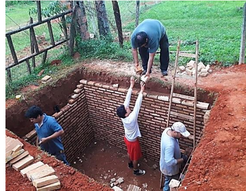
Pastor Miguel and his crew are diligently working on the new septic tank for Barrio Parque Church. The previous was destroyed during torrential rains.
