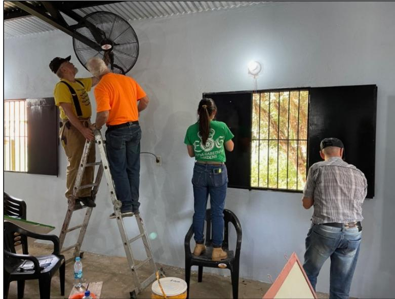
Project Paraguay paid for the walls to go up and the ceiling to be put in. This is the team hard at work. We painted the exterior, interior, floor. We installed electricity, lights, fans, doors, and windows. We also had 5 truckloads of dirt delivered onto the land so as to level the area.
